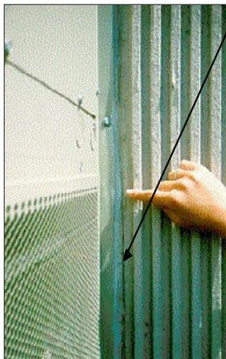
Liquid-applied sealants rely on adhesion. Adhesion is weakest in tension. As structures expand and contract with thermal changes, liquid-sealants eventually separate from substrates.
